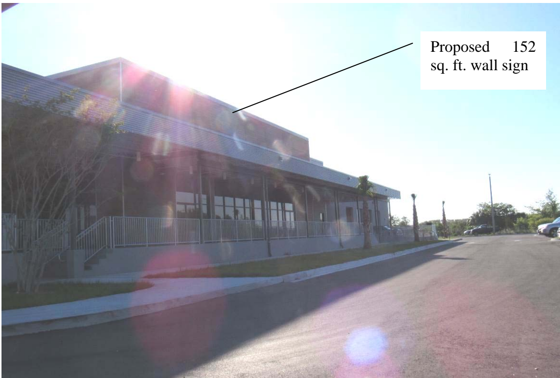
View of existing building
