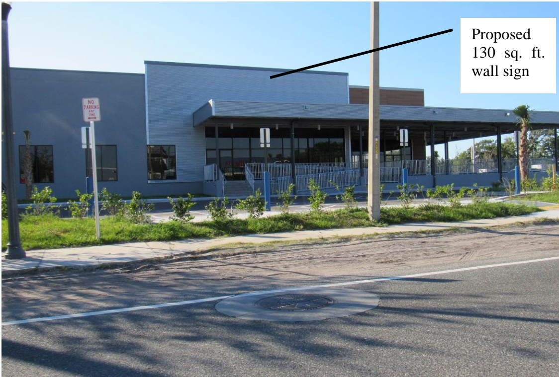
View of existing building
